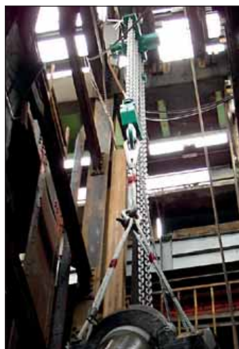
JDN Air Hoist PROFI 37 TI mounting a pipe string in a shaft. At the end of this work the PROFI hoist has to position a 1000m long string with a total weight of 30ton.
